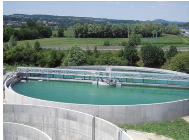
WASTE WATER PLANT Bourgoin-Jallieu (Isère, France)
