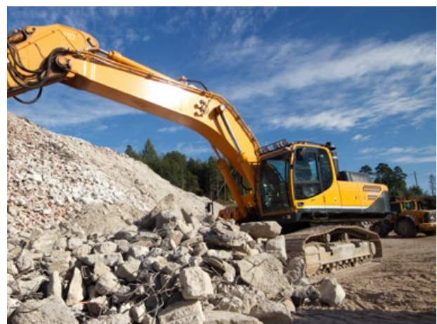
VALORISATION OF RECYCLED AGGREGATES FROM DECONSTRUCTION
