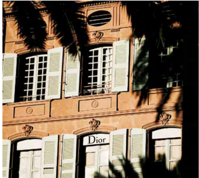
RESTORATION OF THE FAÇADE OF VILLA DE L'AMBASSADE, A DIOR BOUTIQUE Saint-Tropez – Architects: LAC – Contractor: Les Ateliers du Paysage
