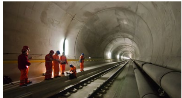
GOTTHARD BASE TUNNEL Zürich, Switzerland
